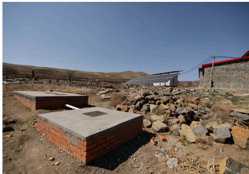
New septic tank at Bobete health center . Photo by Justice Kalebe / PIH
